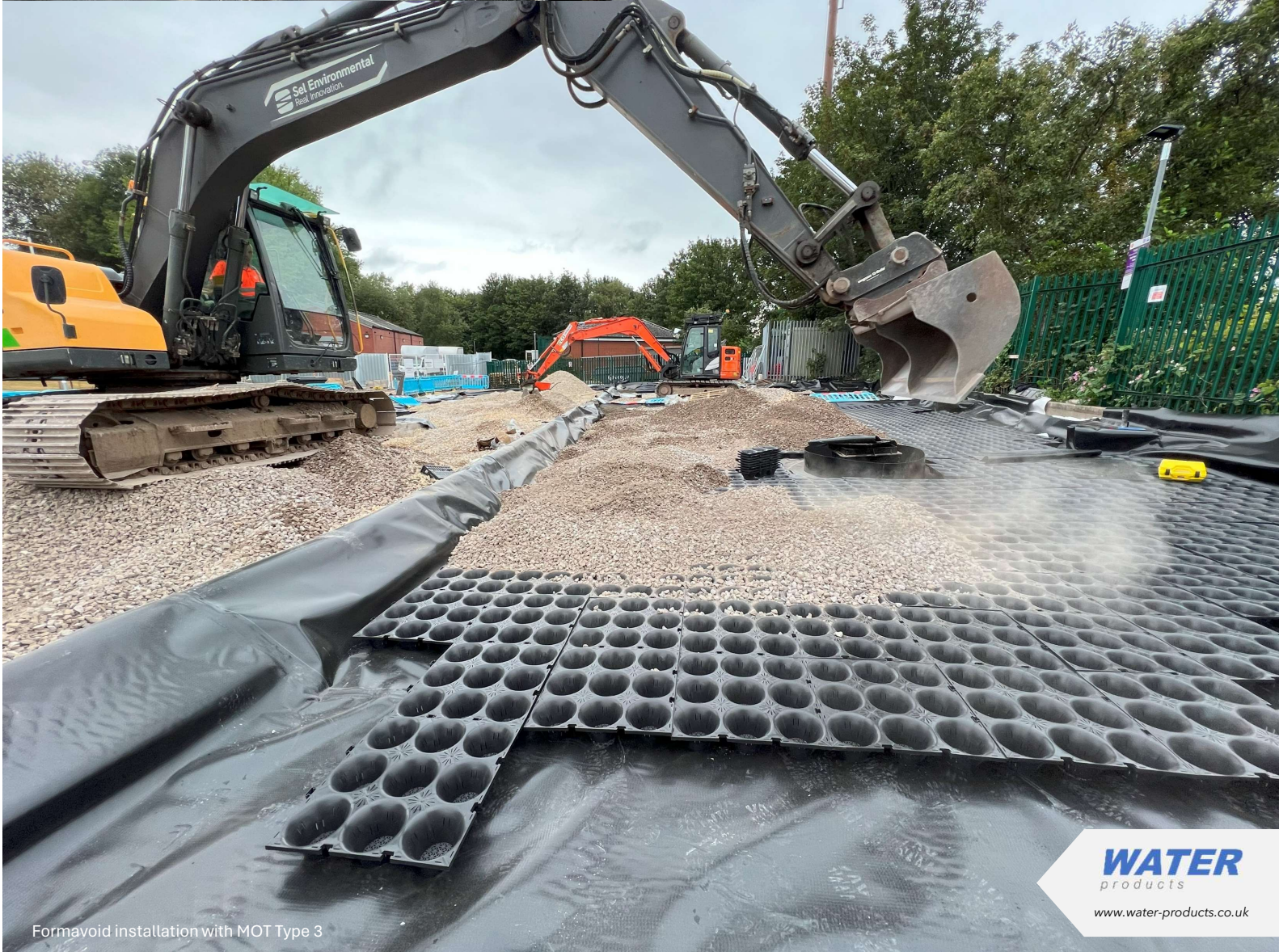
Geomembrane installation & sealing to chambers
