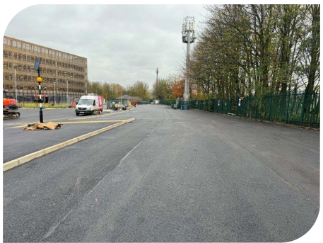
PCC kerb checkdam
